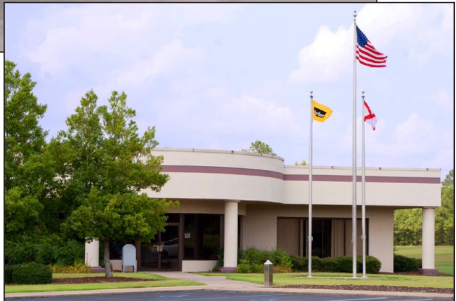
Jacksonville, Alabama, USA
